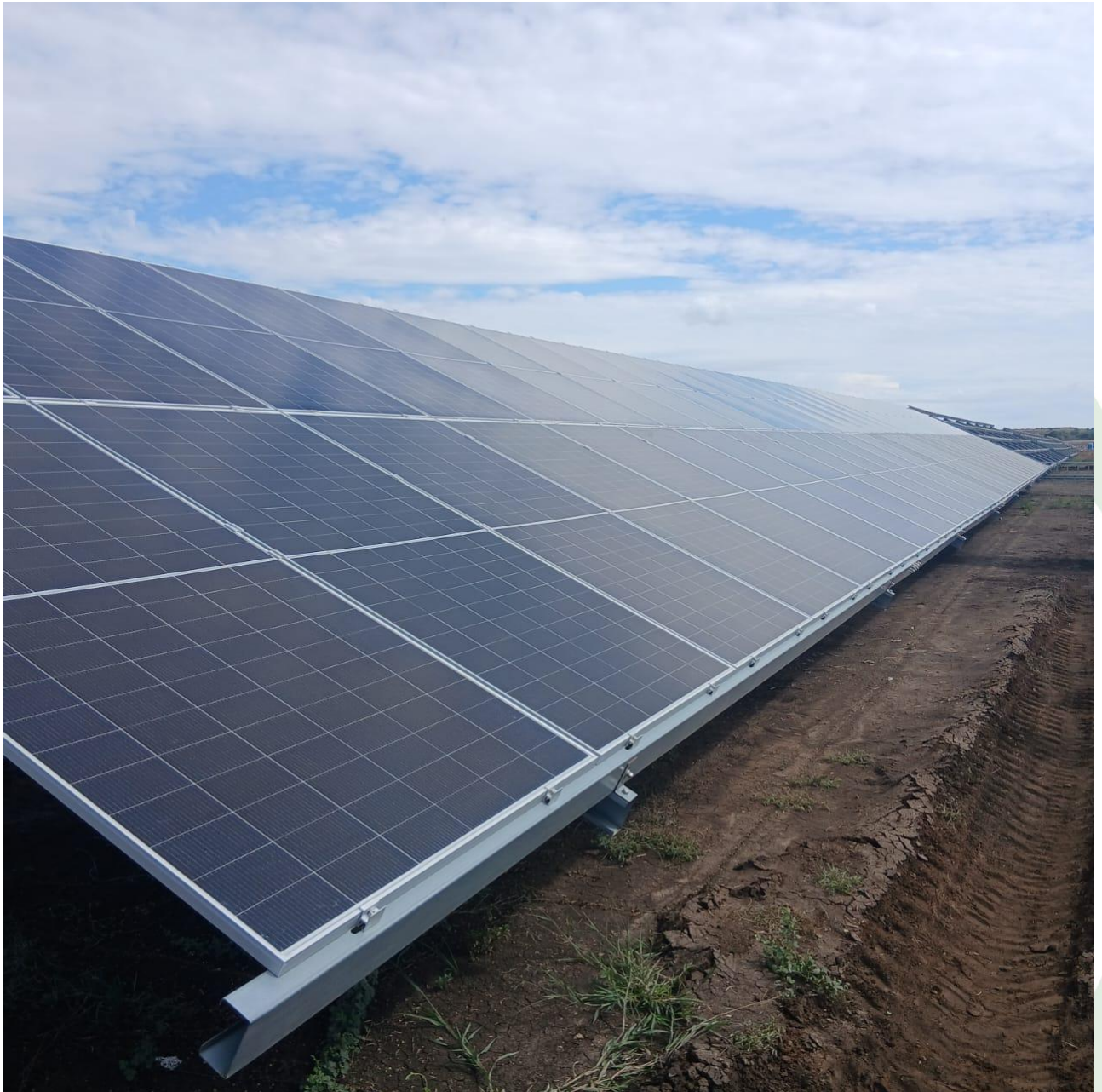
Aluminium clamps are used to secure the panels to the tables.
